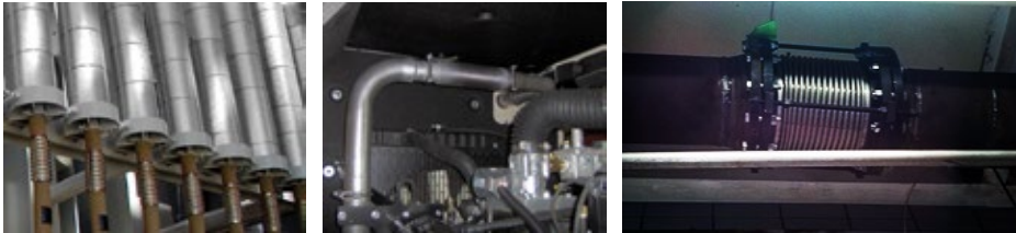
Lined Metal Expansion Joint
